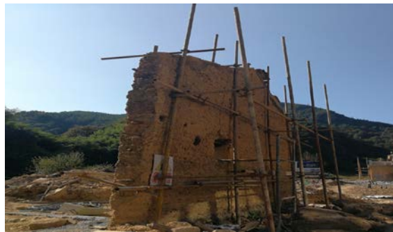
Fig.6 The original oil rammed earth wall of hermit village.
