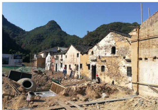
Fig.7 The original rammed earth house village group in the reclusive village.
